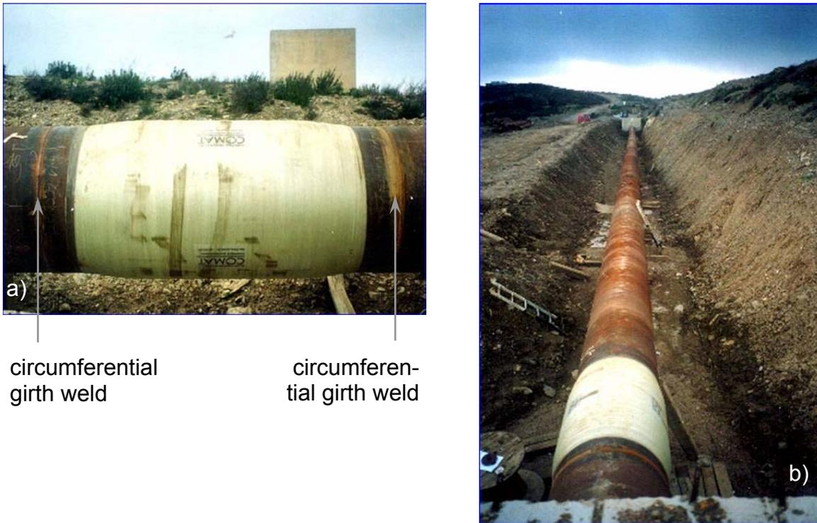
Figure 8: Fibre-reinforced pipe segment following the wrapping process and integrated into the test line (full-scale test)
